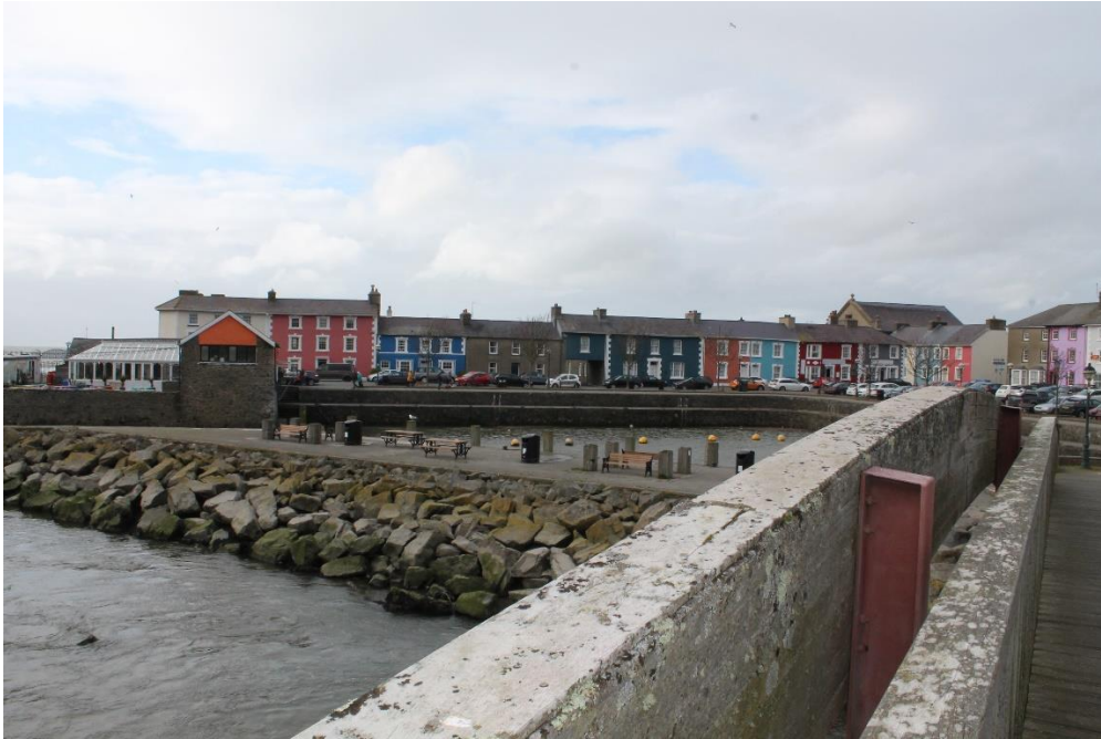
Viewpoint 5 – View of Pwll Cam from Pedestrian footbridge
