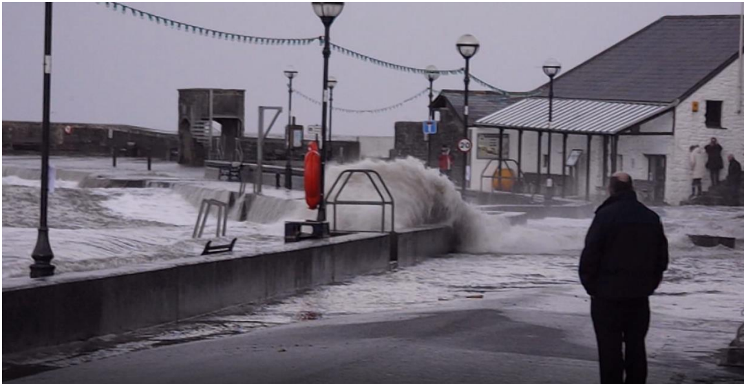
Figure 1 Flooding along Quay Parade
