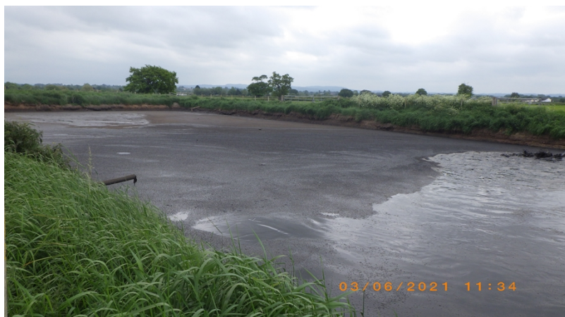
Photo showing digestate lagoon
