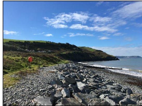
Figure 1-4 Rock Revetment along South Beach
