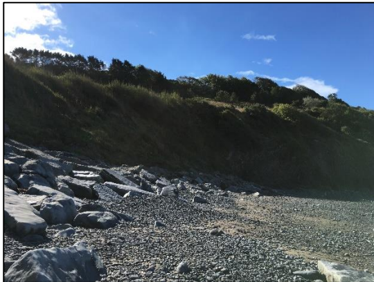
Figure 1-3 Eroding Cliff on South Beach
