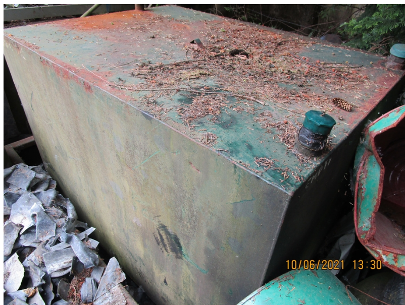
Figure 2. Double bunded tank used to store motor oils.
