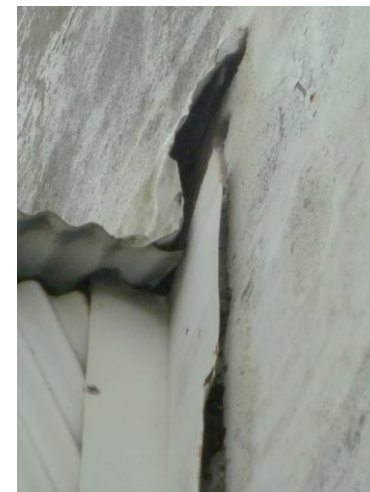
Plate 10: Gaps between Conveyor Enclosure and Transfer Tower
