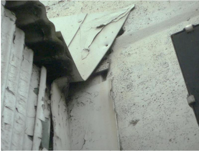
Plate 11: Gaps between Conveyor Enclosure and Transfer Tower
