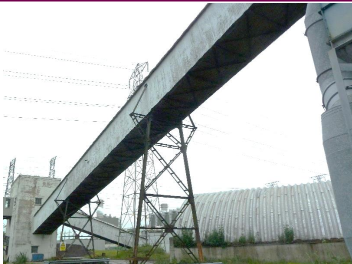
Plate 19: Gaps between Conveyor Enclosure and Transfer Tower
