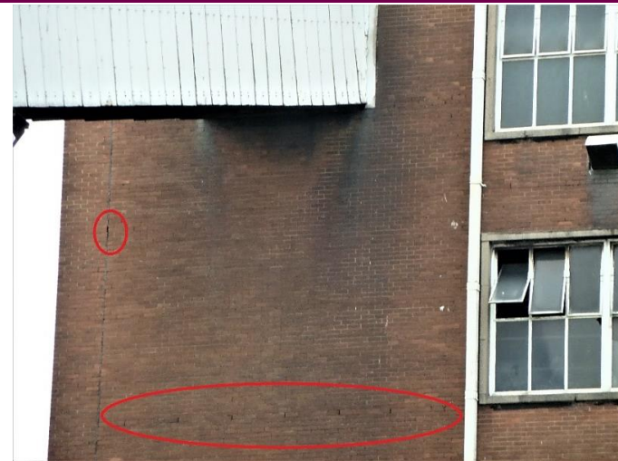
Plate 14: Gaps in the Bunker Hall Brickwork
