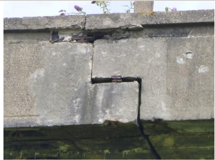
Plate 2: Flyover Bridge Expansion Gap
