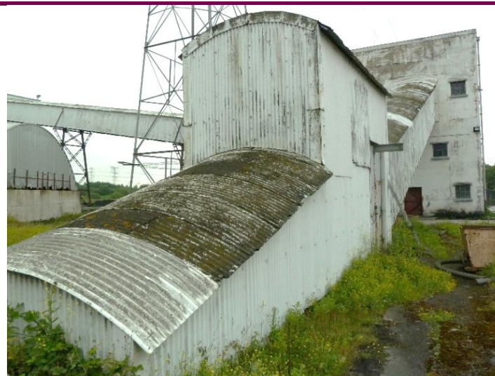
Plate 20: Example of Enclosure where Conveyors Go Below Ground
