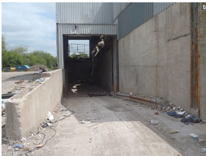
Ramp cleared of waste
