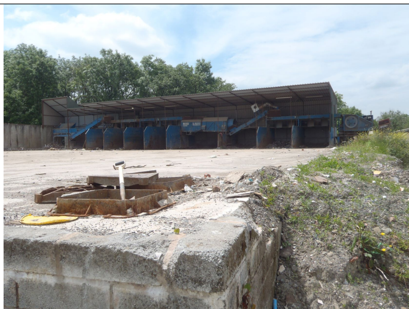
Outside impermeable surface cleared of soil and stone contaminated waste
