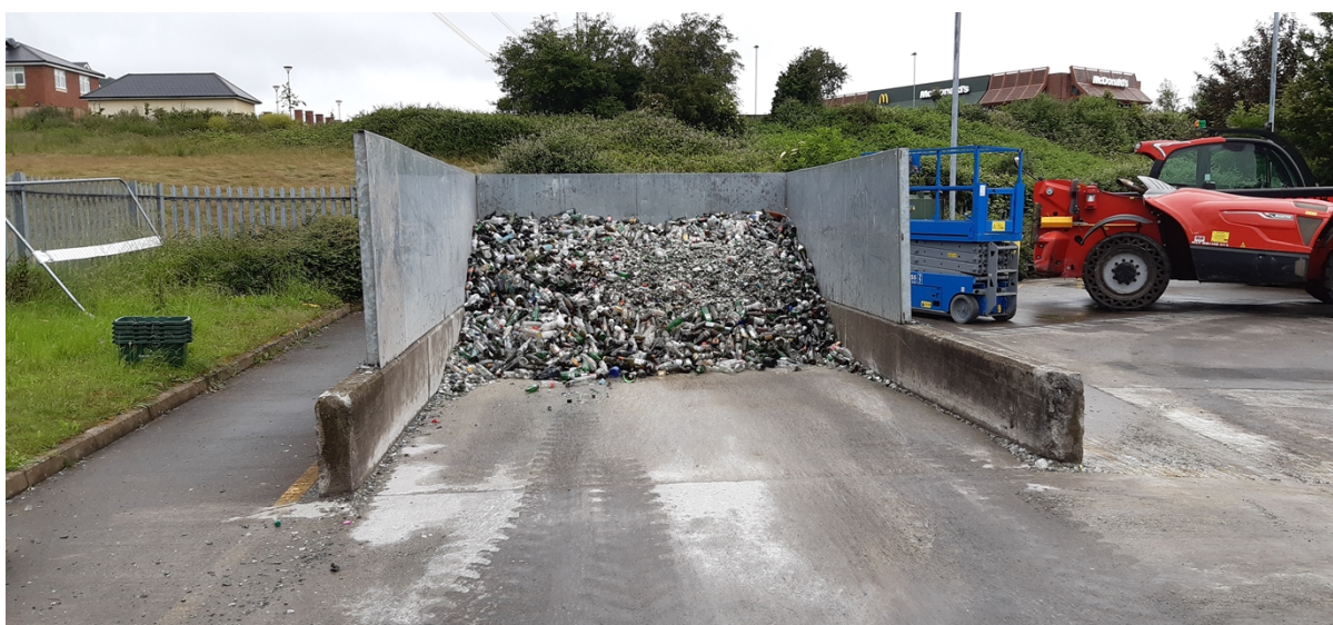
Photo 8 - Waste Transfer Station section holding various waste streams within outside
