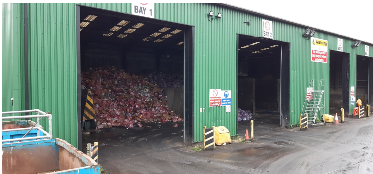
Photo 6 - Waste Transfer Station section holding various waste streams within covered housing
