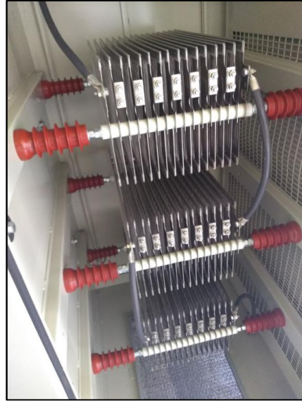
A380 NERs & Supporting Brackets - Defect Free
