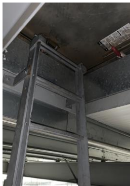
Image 8 showing access locked access hatch
