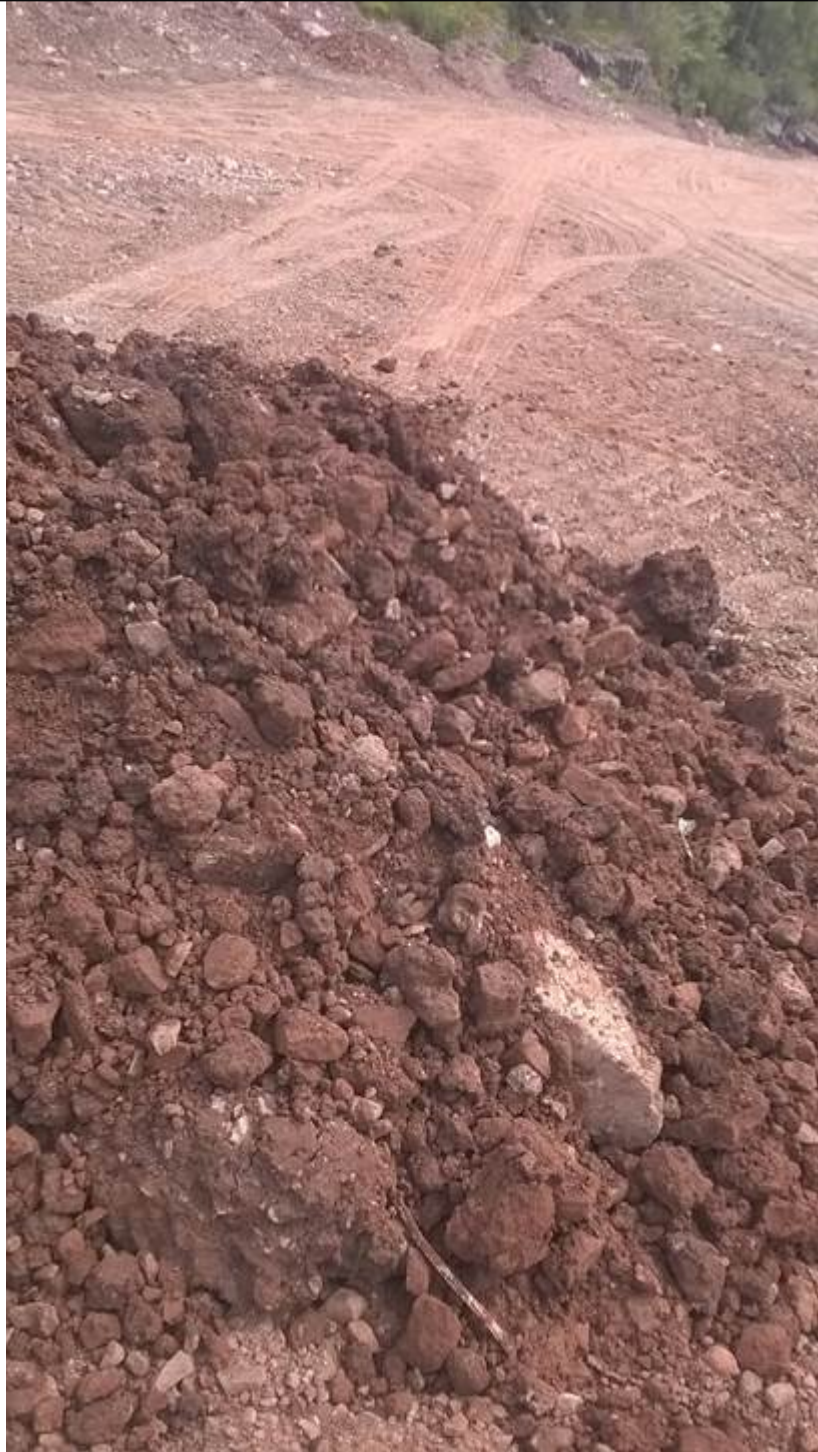
Pic 2 above – Shows the latest offload comprising stones and red mud. Occasional concrete fragments were present which fitted the sites permitted material list.
