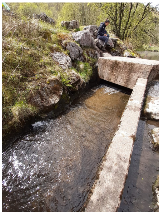
HEP intake looking upstream.
