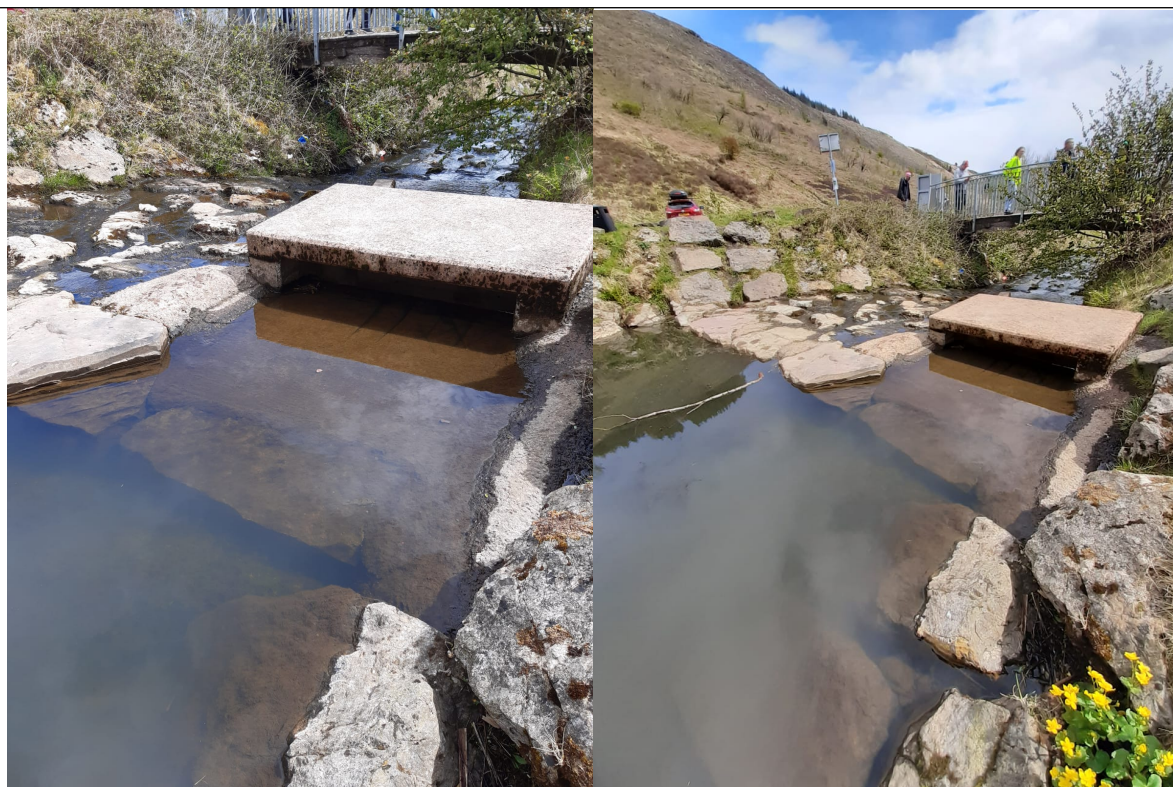
Intake weir looking downstream. Screen under concrete cover.
