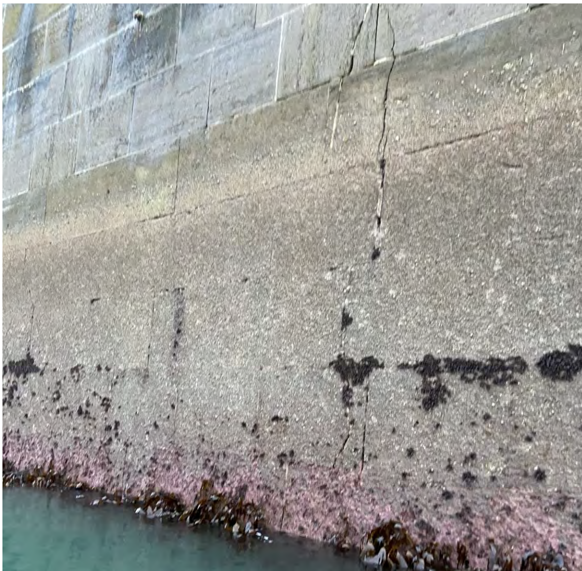
Plate 8 Evidence of cracking within the main bullnose structure above the waterline observed during ROV inspection transect.
