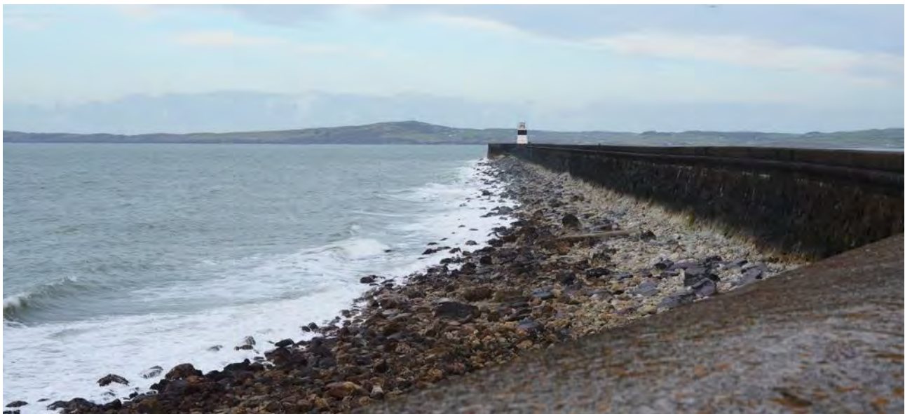
Figure 2 Holyhead Breakwater at low tide exposing the seaward rocky base
