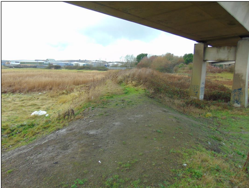
Plate 16: Flood defences on the eastern bank of the River Rhymney beneath the A4232. View to northwest.
