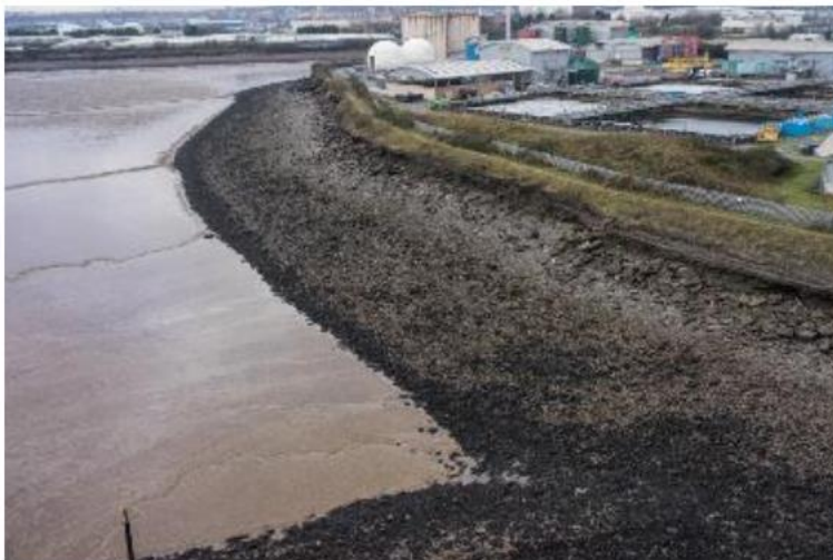
Figure 4-3: Steep ridge to the west of the River Rhymney, containing coarse waste materials
