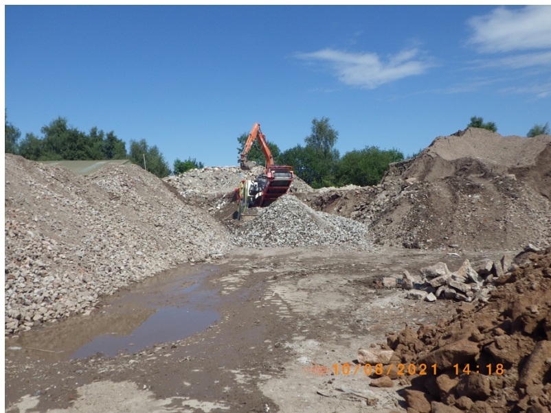
Photo 6: Inert storage area
