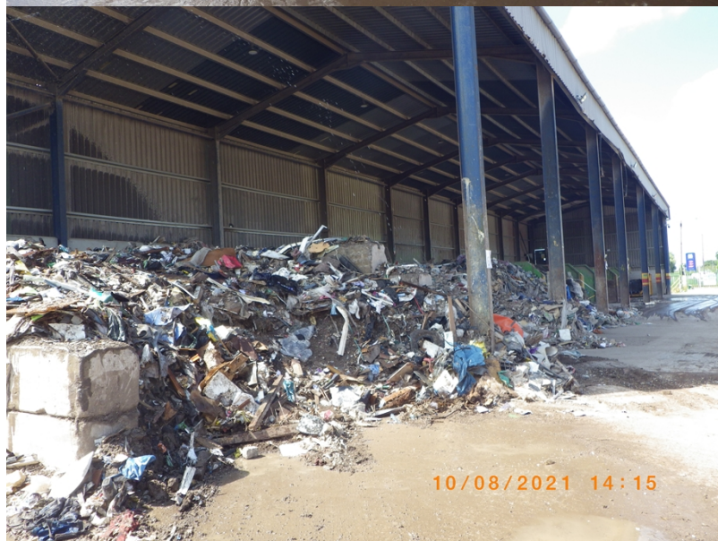
Photos 1 & 2 of transfer building which contains Household, Commercial & Industrial waste
