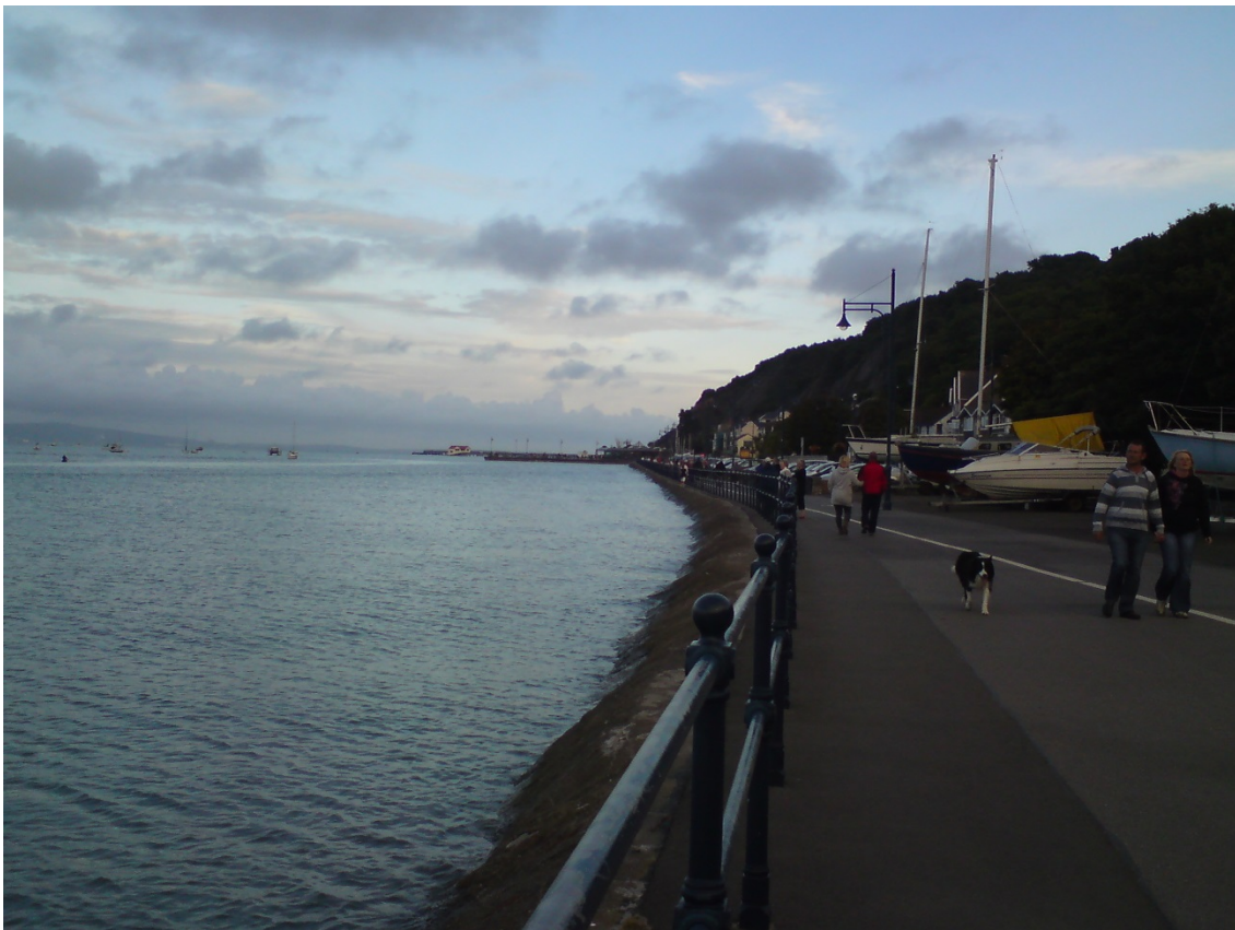
Figure 14. Small magnitude wind generated waves along Mumbles frontage, despite southwesterly waves of heights in excess of 1 m off Mumbles Head (Figure 15)
