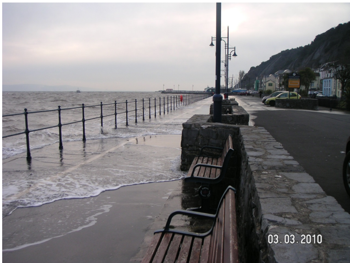
Figure 16. Overtopping events throughout defence sections on 03/03/2010, where wave conditions were from a southeasterly direction (Figure 17)
