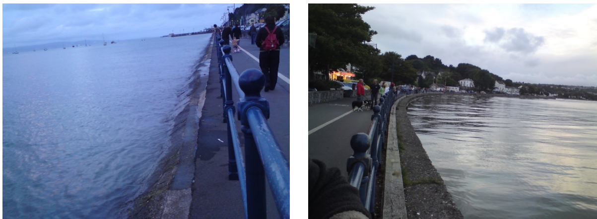
Figure 9. Calm conditions throughout Mumbles defences at near HAT levels on 09/09/2010
