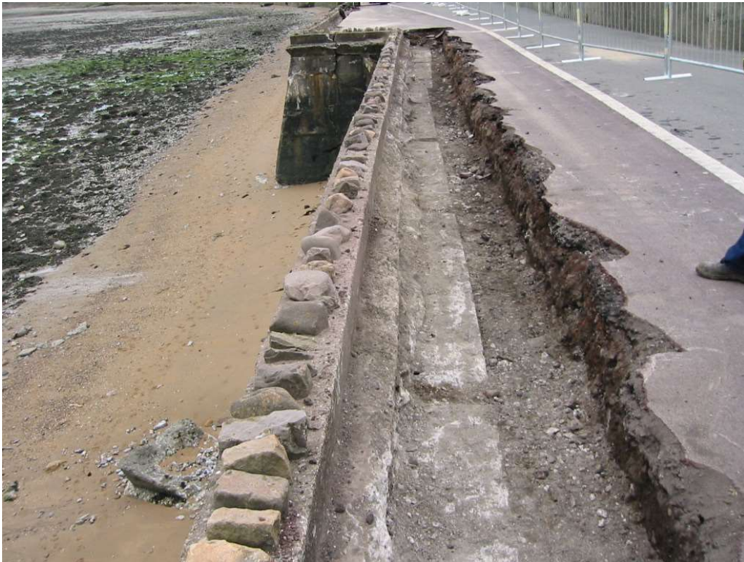
Figure 1 - Photo from hand rail construction in 2002
