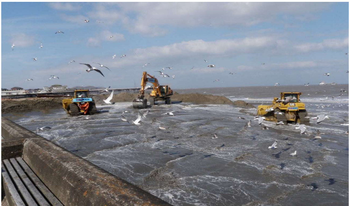
Photo 4.4: Beach recharge works during previous phase – plant movements in the intertidal area
