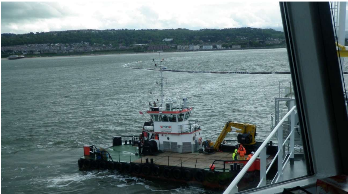
Photo 4.2: Beach recharge works during previous phase – view from TSHD of the floating pipeline
