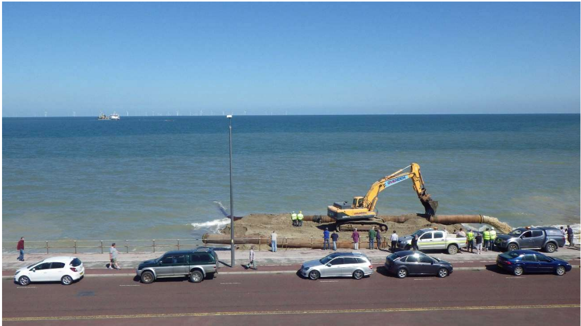
Photo 4.3: Beach recharge works during previous phase – view from shore of the sinker and shore pipelines with the TSHD and floating line in the distance
