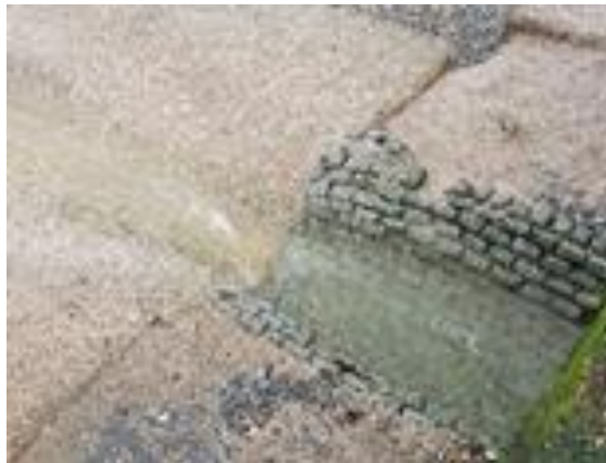
Figure C.4: Running Water (culverted)
