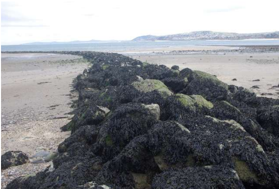
Figure 3.16: Curved groyne adjacent to the harbour
