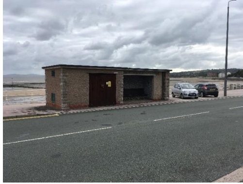
Figure C.2: Buildings and Infrastructure
