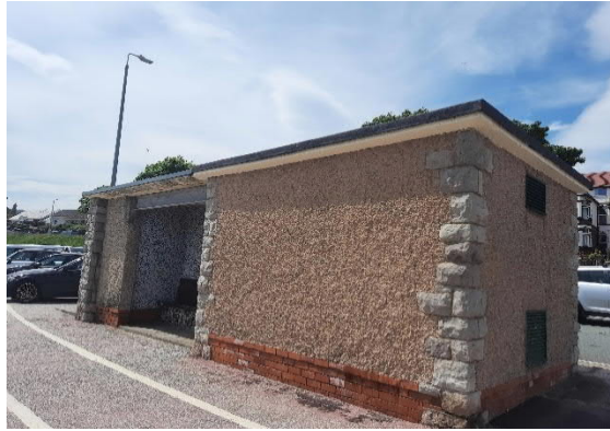
Figure A.2: Seating shelter and energy networks building (B2)
