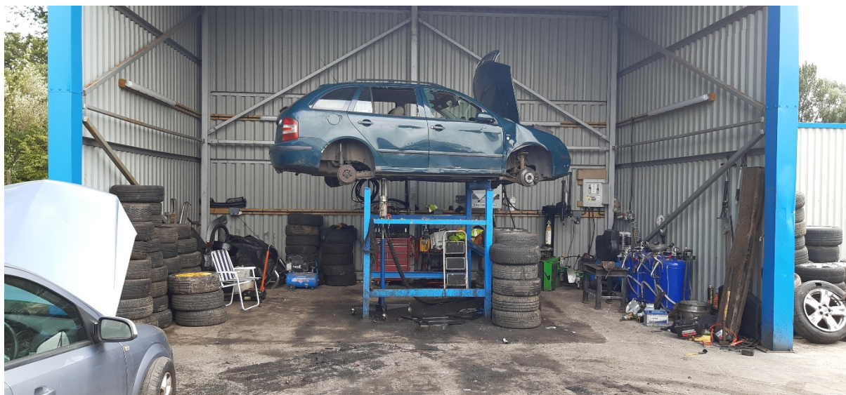
Photo 7 - Fully operational ELV depollution bay
