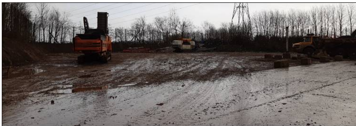
Image 9 - showing the SRF area cleared of all material, taken 16 February 2021
