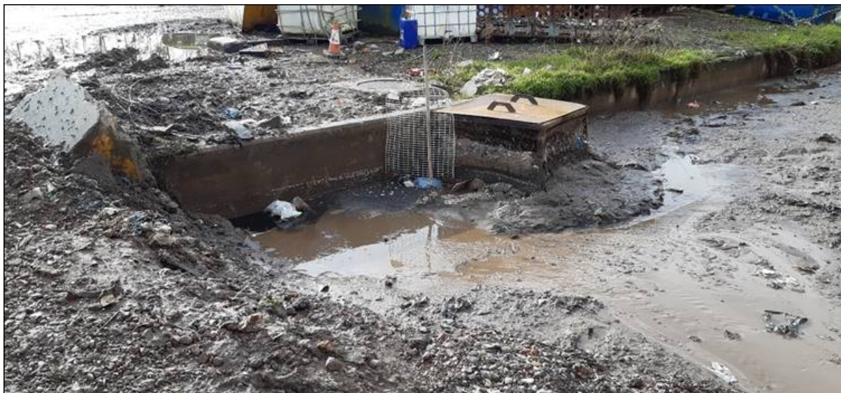
Image 10 – showing the drain entry on Field 1, taken 16 February 2021
