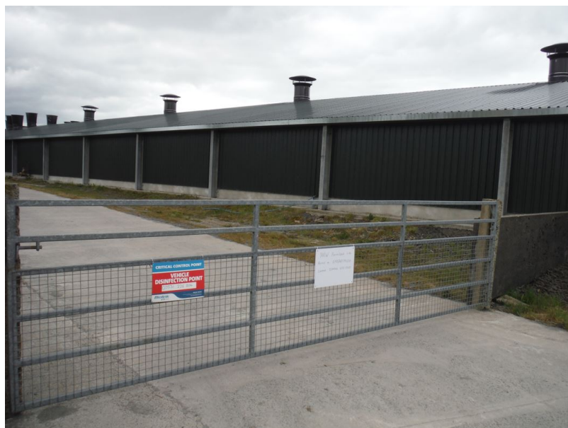
(Above) Temporary ID board on access gate.
