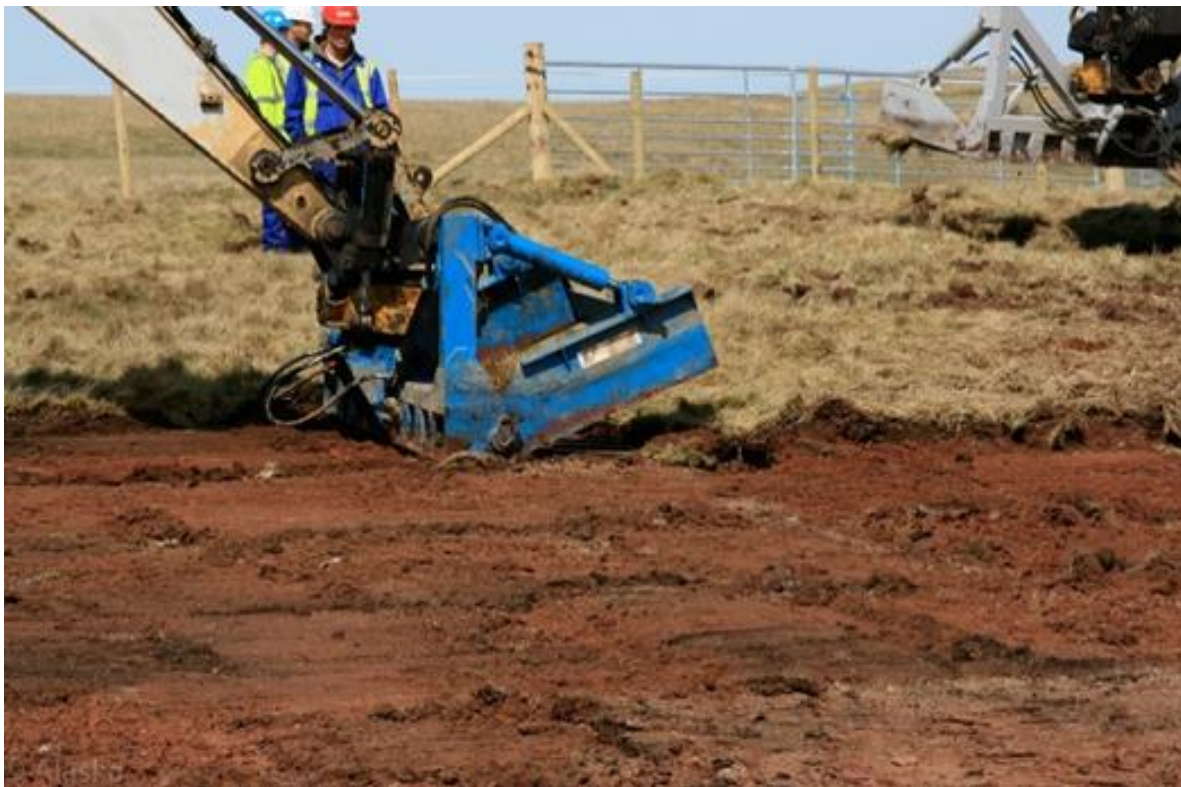
Figure 3-1: Mechanised harvesting of vegetated turf
