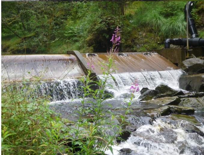
Photograph 1: Point of abstraction 02/06/2021 11/08/2021
