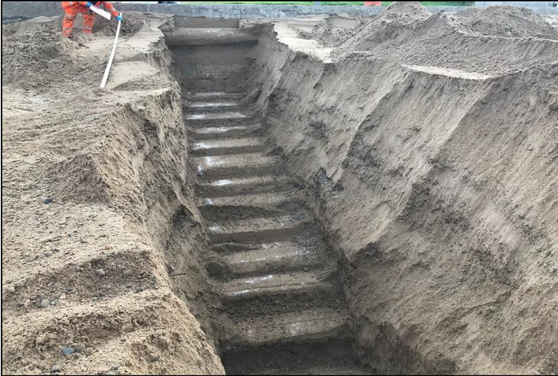
Figure 2.4: Existing buried stepped revetment
