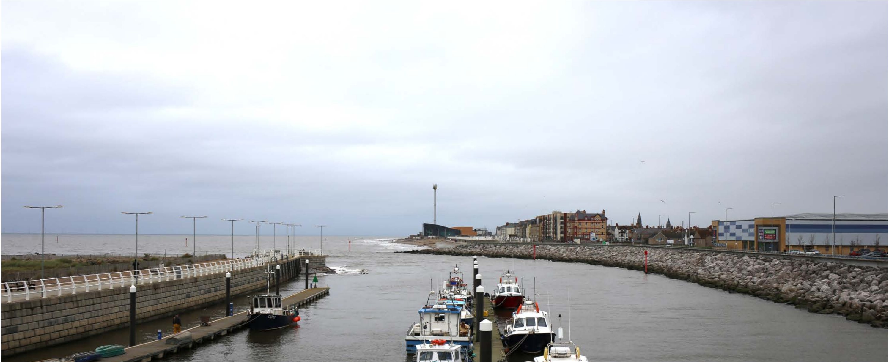
Viewpoint 9 Pedestrians on Pont y Ddraig Bridge
