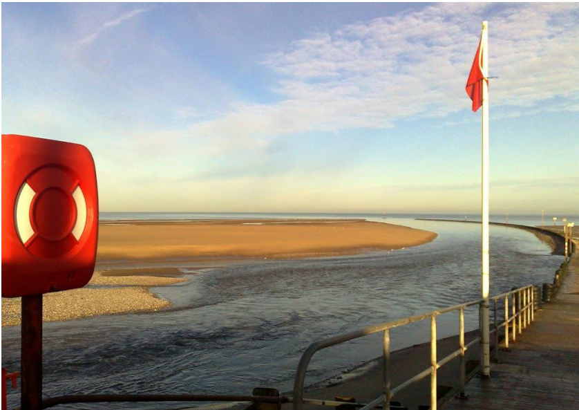
Figure 5.14: River Clwyd training wall shown below is included in the coastline evolution model as a groyne, to ensure its sheltering effect is considered in the longshore transport rates.
