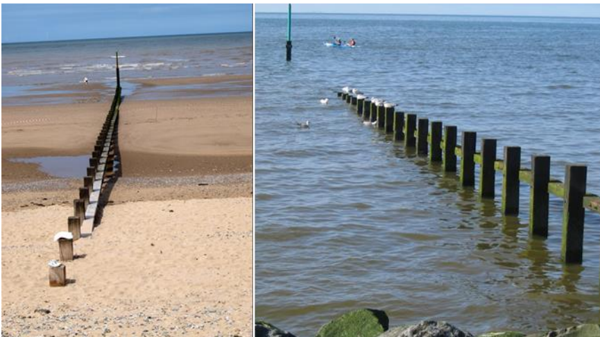
Figure 5.15: Example of the wooden groynes located in Central Rhyl frontage.
