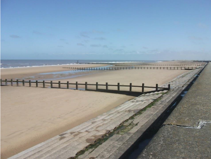
Figure 5.16: East Rhyll wooden groynes field. Please note the structures condition and how the sediment is entirely retained by the structures. The image also shows the concrete stepped revetment maintaining the coastline position.
