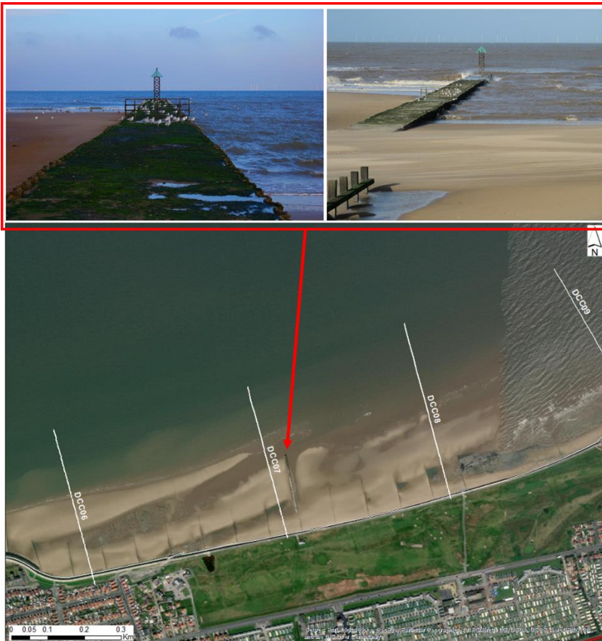
Figure 5.17: East Rhyll concrete rock groyne blocking part of the sediment transport. The structure is included in the coastline evolution model.
