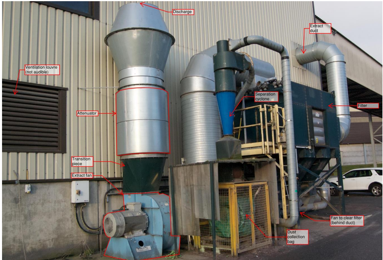
Figure 1-2 – Annotated photograph showing stages of air extraction and dust separation
