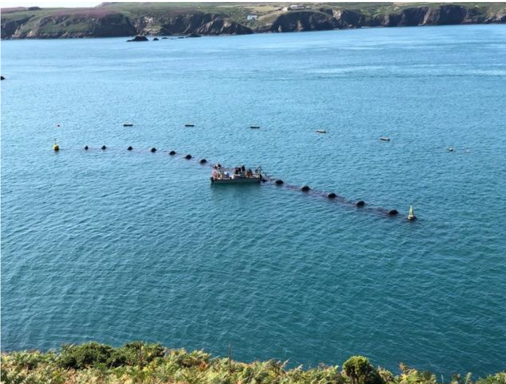
Figure 5 a/ Powered pontoon launching from St Justinians. b/ Carn ar Wig trial site being worked on.
