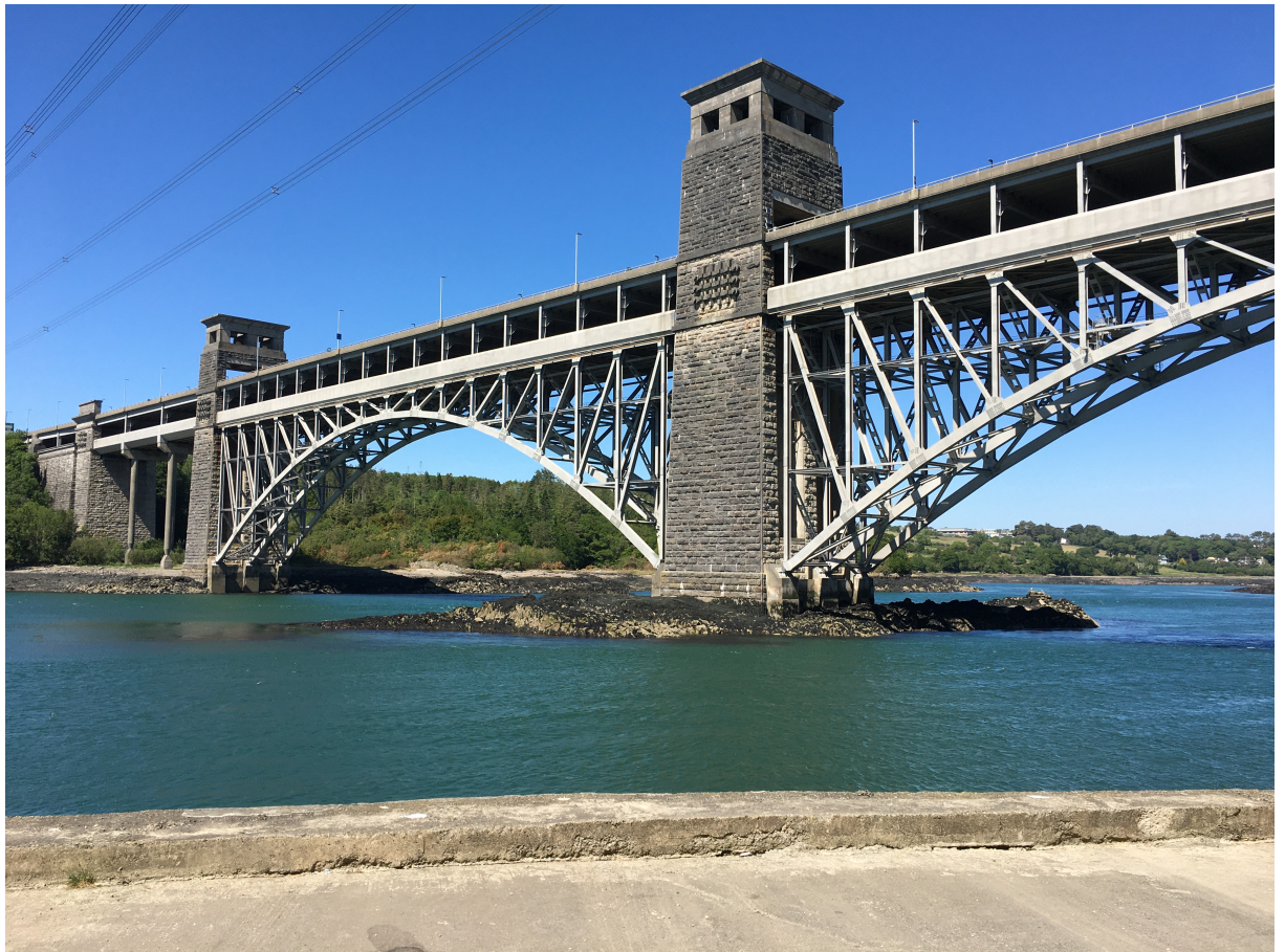
Photo showing tower where access will be cantilevered out from openings off steelwork either side of the stonework from the rail service road (level with the decor stone). Then bridged between both across the decoration with a stair tower extended off to one of the window openings.
