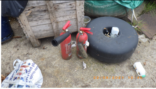
Fire extinguishers on site
