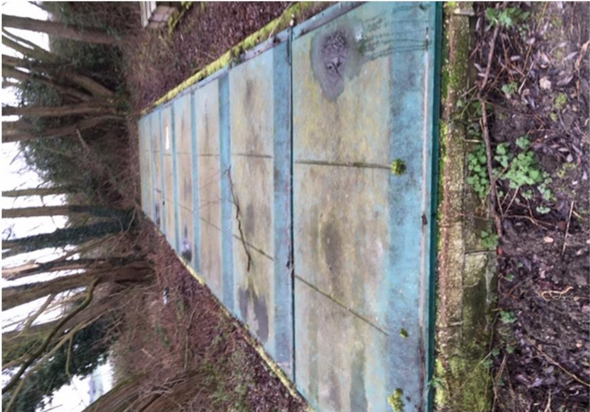
Photo 1: Primary Settlement Chamber (below grass) – Liquids pumped over to 2 nd chamber (below grass) – Liquids pumped to Secondary Treatment System via over ground pipe network
