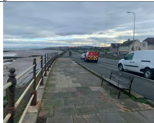
Photograph 10. Road/pavement on south of site
