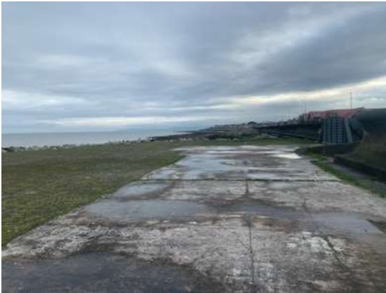
11 Hardstanding in east of site.
