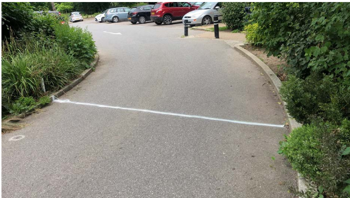
Figure 16 – Surface coil secured to road with survey nail & highlighted with spray paint if required.
