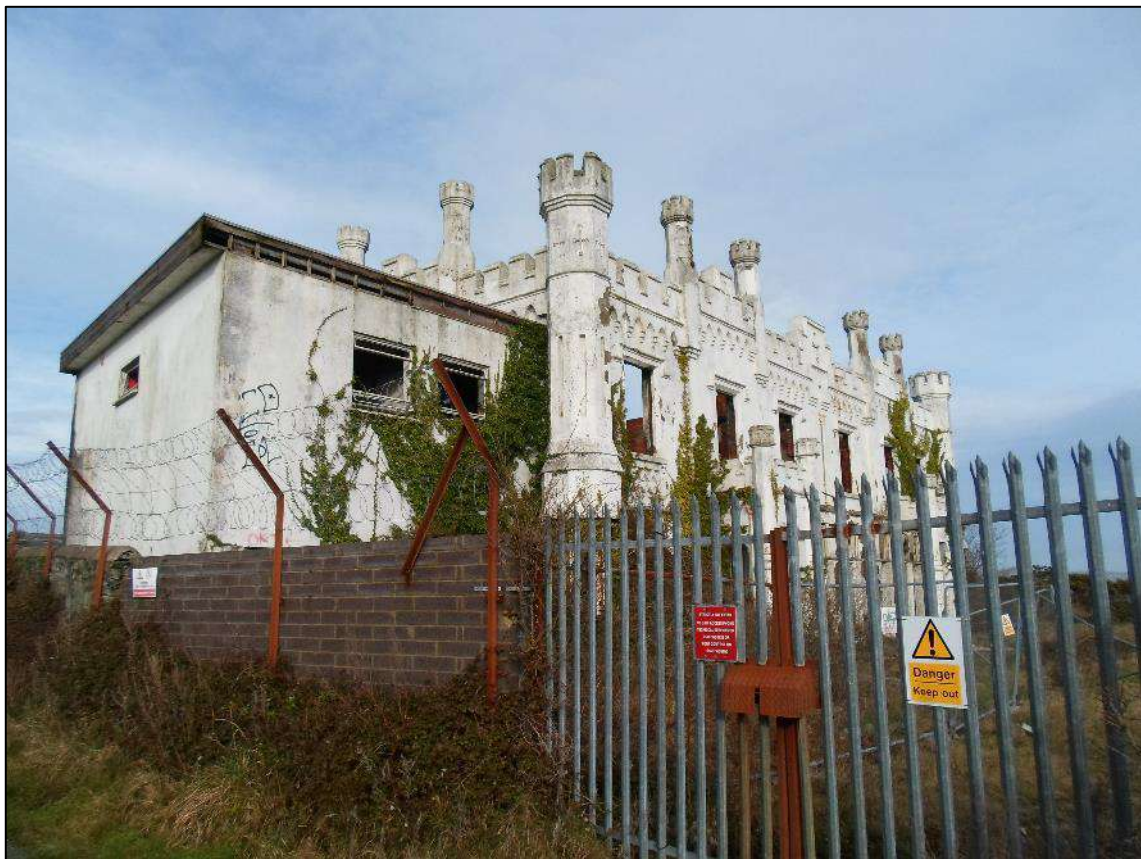
Plate 2. Soldiers Point House (LB 14760), looking north
