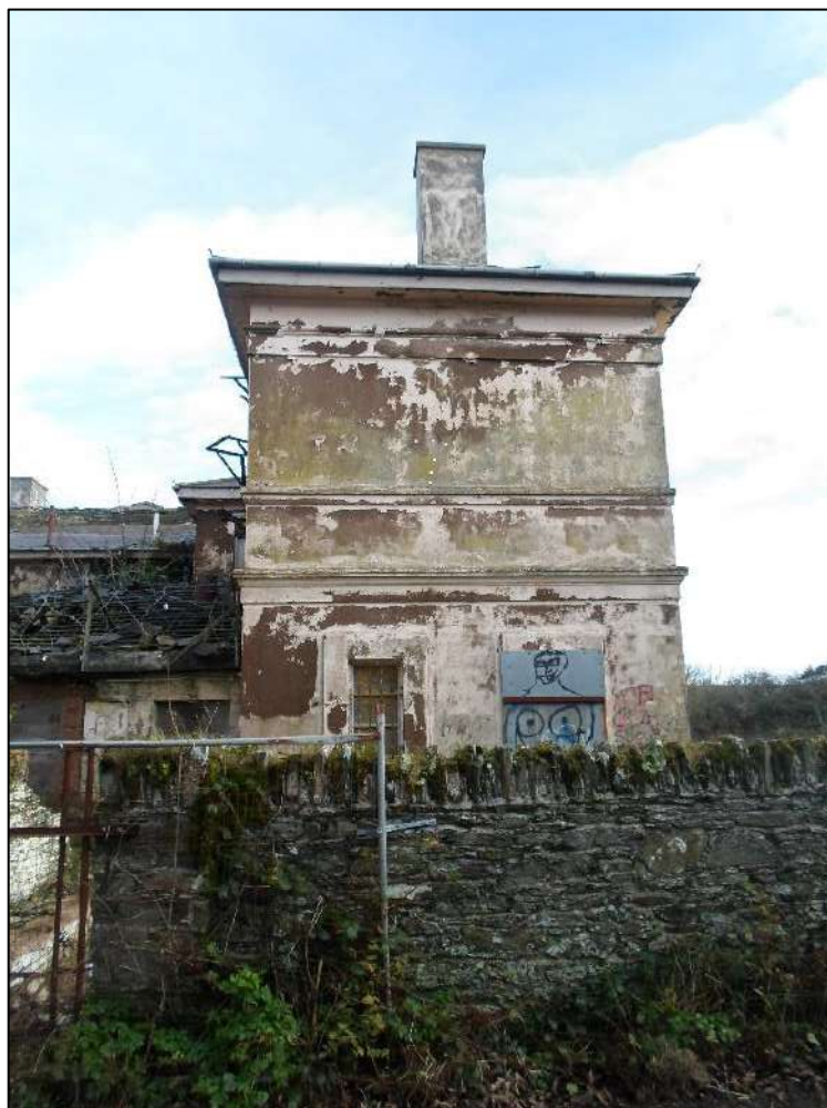
Plate 14. Porth-y-Felin House (LB 14759), looking north-east
