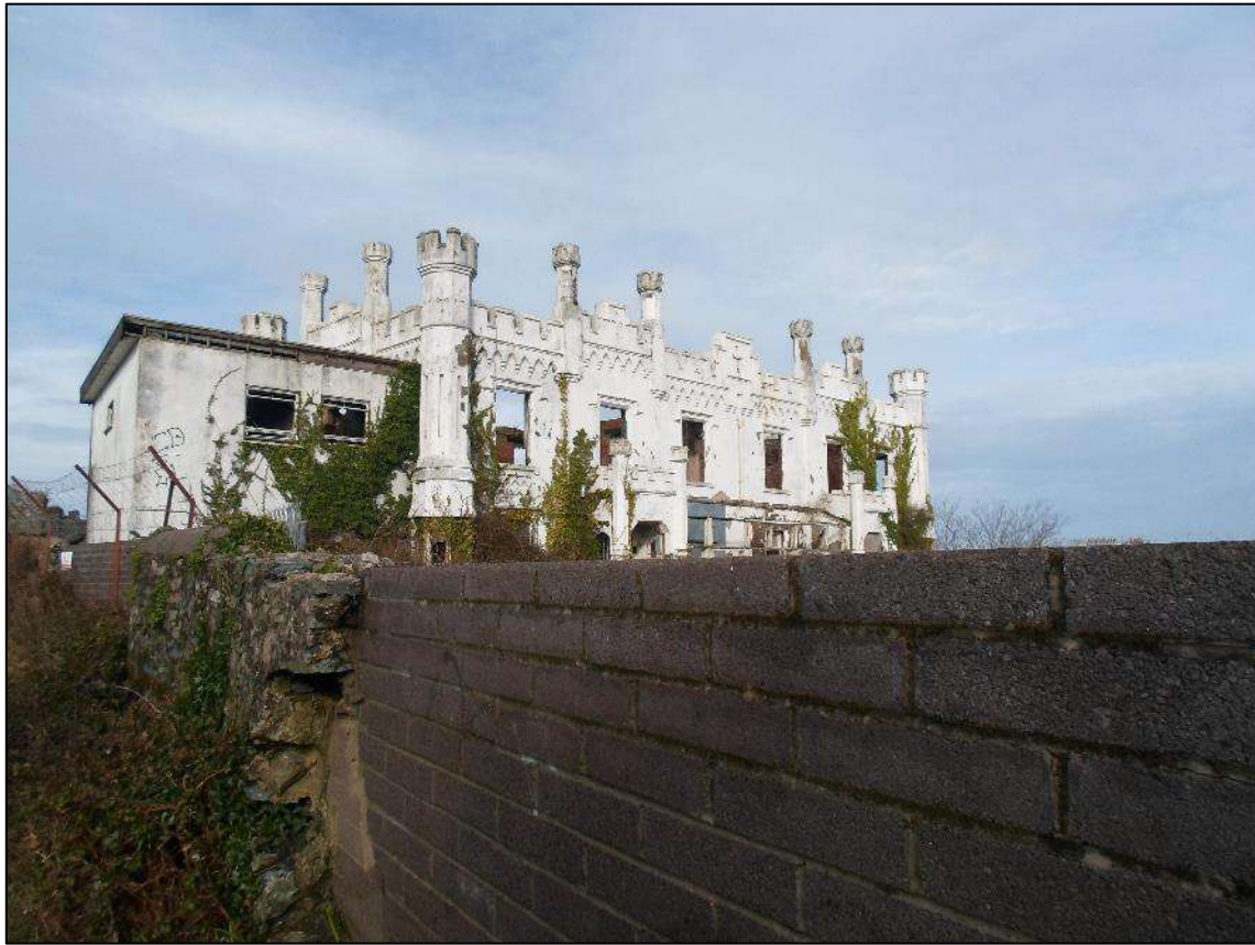
Plate 1. Soldiers Point House (LB 14760), looking north
