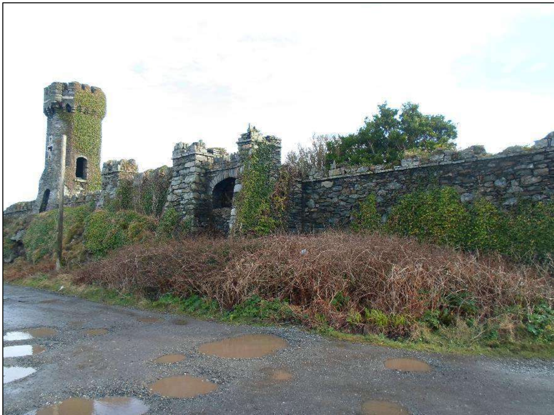
Plate 10. Screen Wall to Soldier's Point House (LB 14761), looking east
