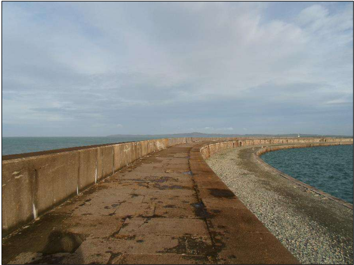
Plate 43. Holyhead Breakwater (LB 5743), looking north
