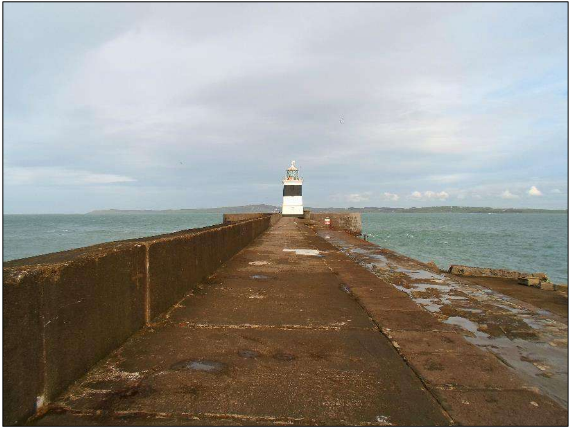
Plate 47. Looking north towards Lighthouse on Holyhead Breakwater (LB 5744)
