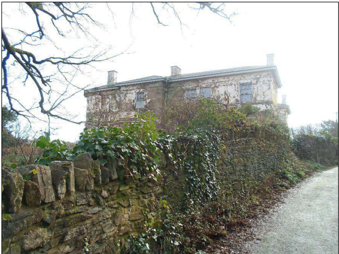
Plate 22. Porth-y-Felin House (LB 14759), looking east
