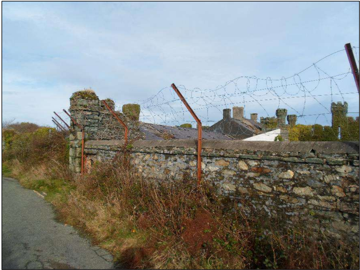
Plate 31. Buildings to rear of Soldiers Point House (LB 14760), looking north
