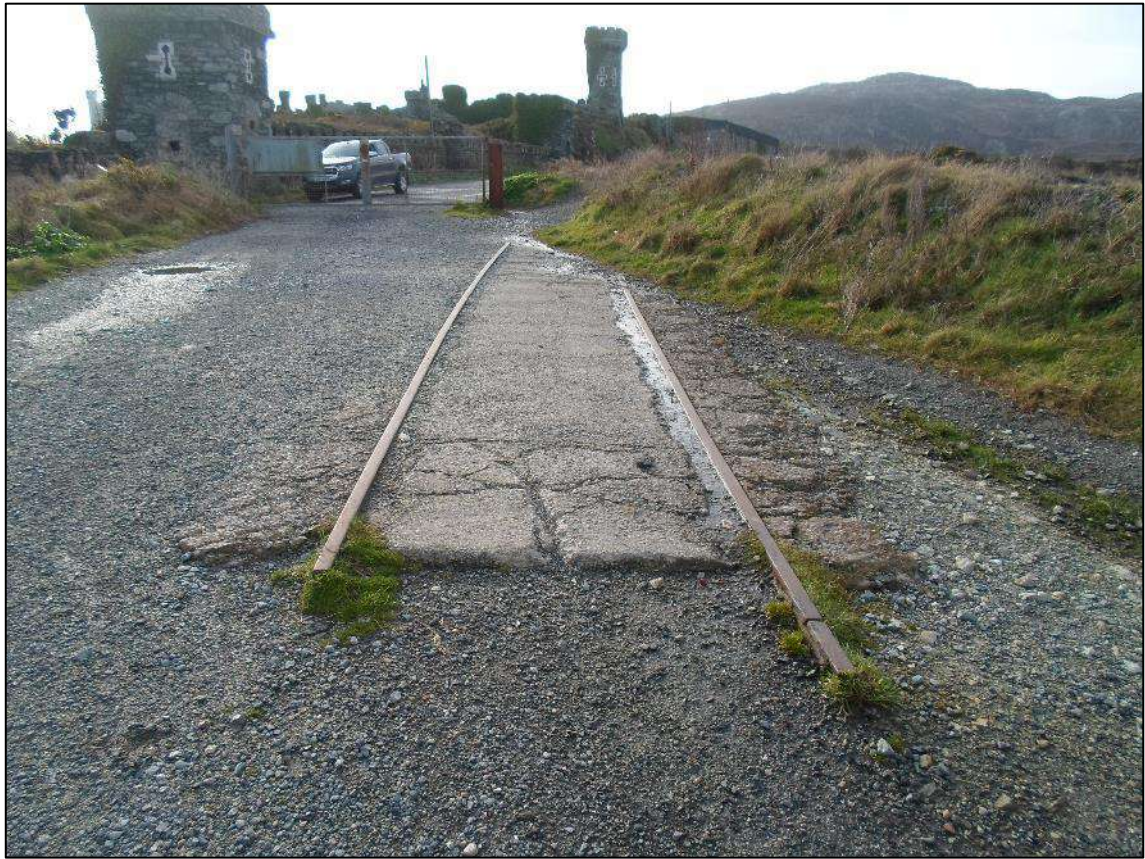
Plate 41. Possible remains of Breakwater Tramway (PRN 16076), looking north-west
