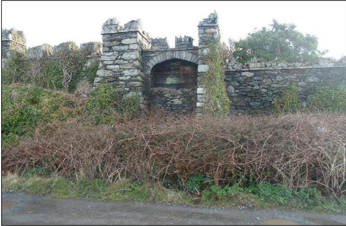
Plate 35. Screen Wall to Soldier's Point House (LB 14761), looking south-east
