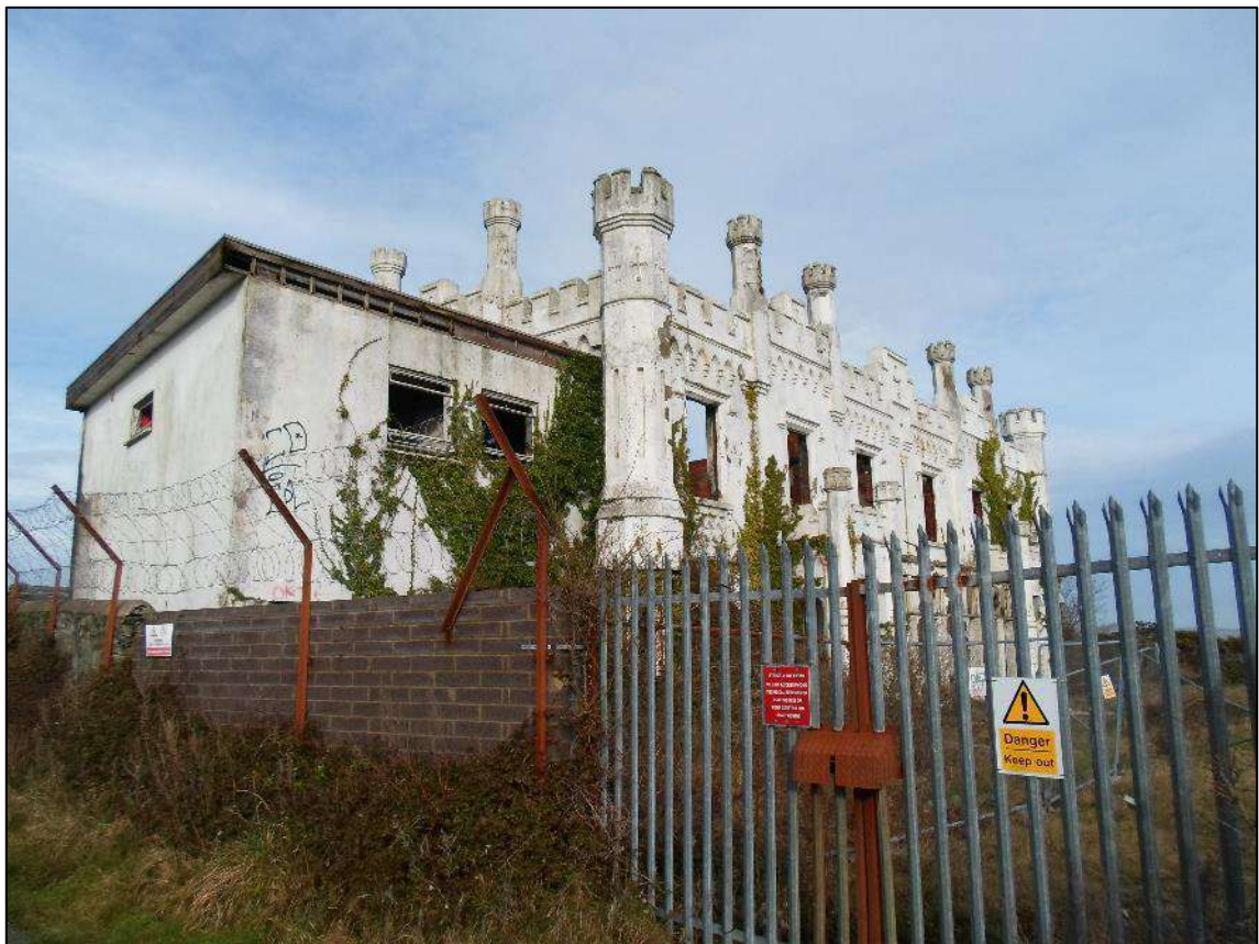
Plate 26. Soldiers Point House (LB 14760), looking north
