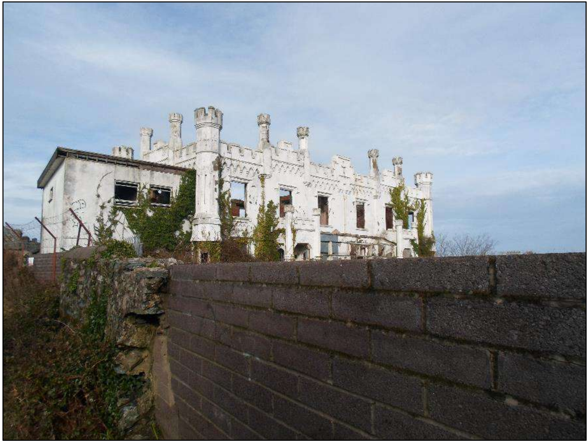
Plate 25. Soldiers Point House (LB 14760), looking north
