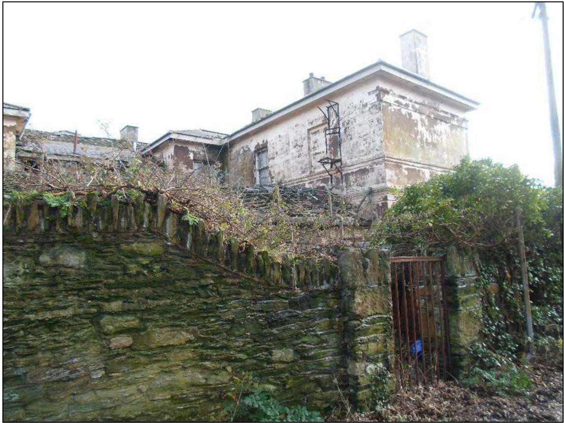
Plate 21. Porth-y-Felin House (LB 14759), looking east
