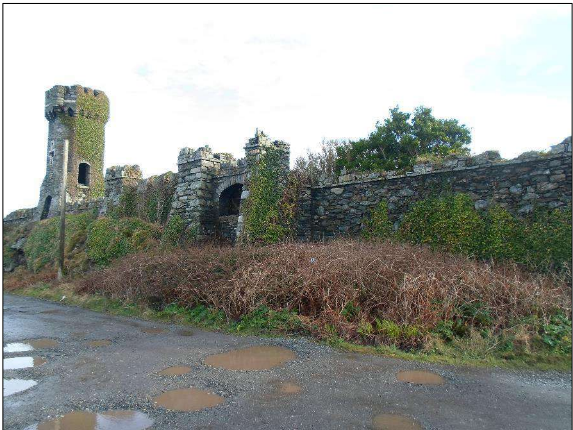
Plate 34. Screen Wall to Soldier's Point House (LB 14761), looking east
