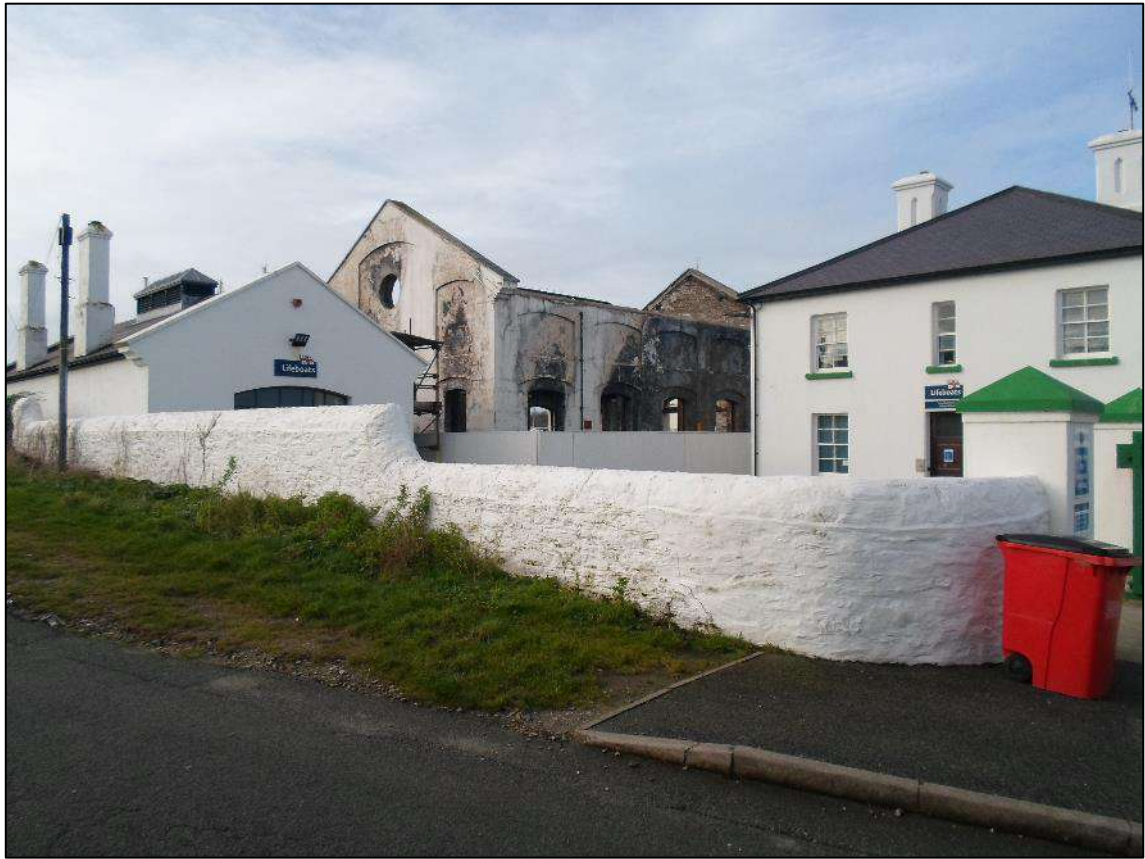
Plate 15. Trinity Yard Small Workshop (LB 14732), Trinity Yard Large Workshop (LB 14731), and Trinity House Office (LB 14730) from boundary of proposed site, looking south-west
