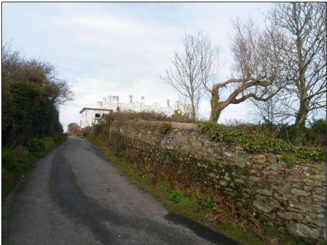
Plate 24. View towards Soldiers Point House (LB 14760), looking north
