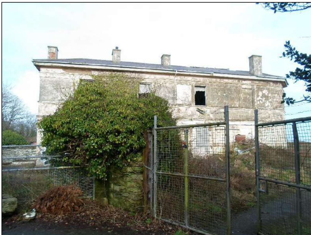
Plate 19. Zone 2 – Porth-y-Felin: Porth-y-Felin House (LB 14759), looking north
