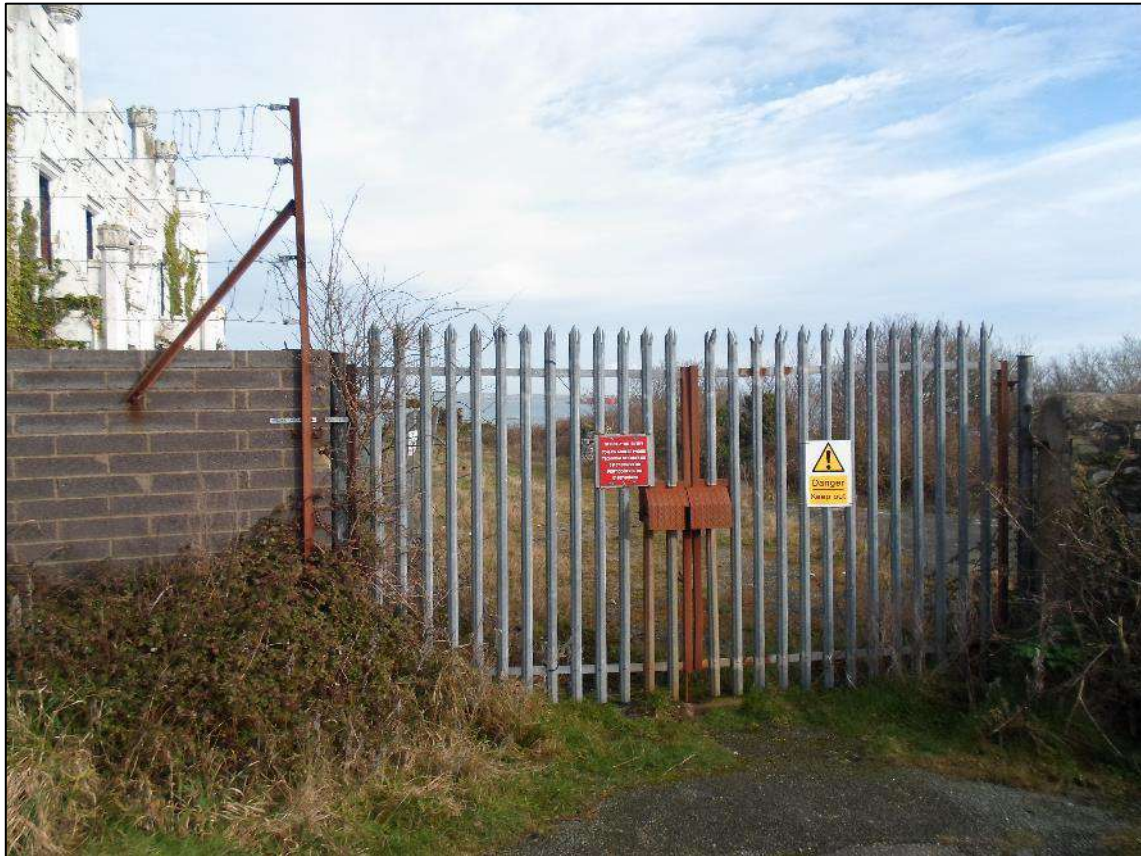
Plate 27. Soldiers Point House (LB 14760), looking north-east towards New Harbour and proposed site
