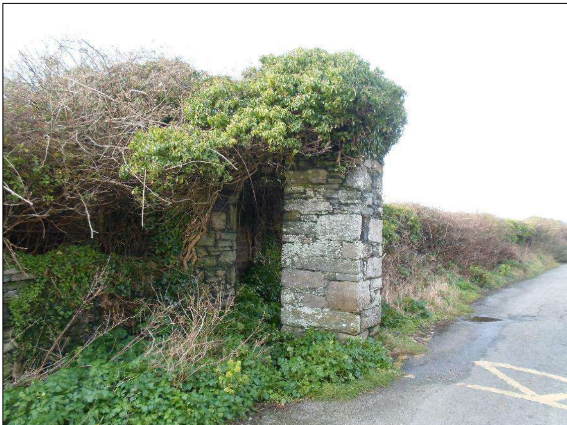
Plate 28. Stone archway opposite Soldiers Point House (LB 14760), looking north-west
