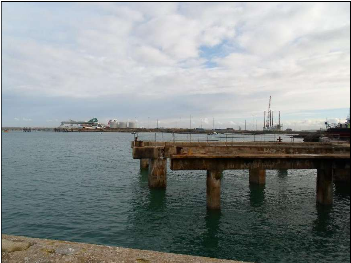
Plate 2. View towards New Harbour from PRN 34023, looking east
