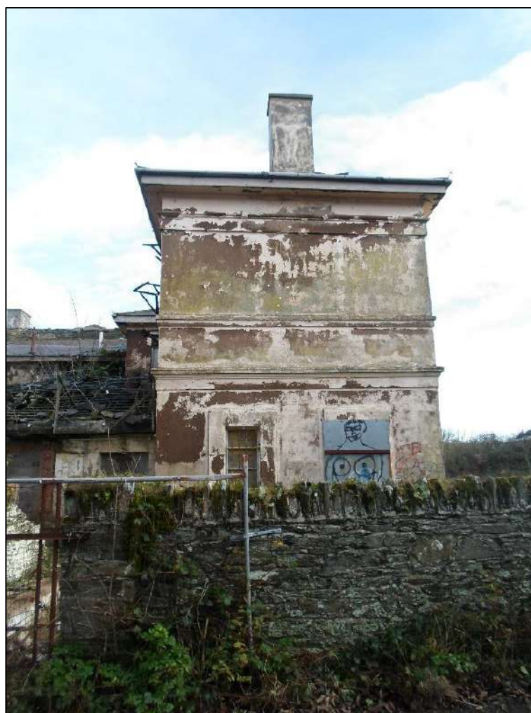
Plate 20. Porth-y-Felin House (LB 14759), looking north-east
