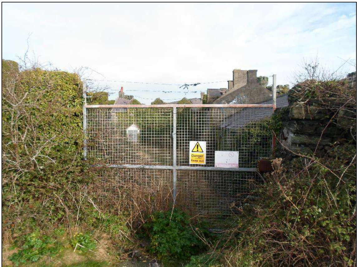
Plate 32. Buildings to rear of Soldiers Point House (LB 14760), looking north
