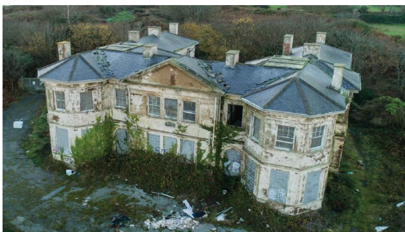
Aerial view of Porth-y-Felin House, demonstrating its current state of disrepair
