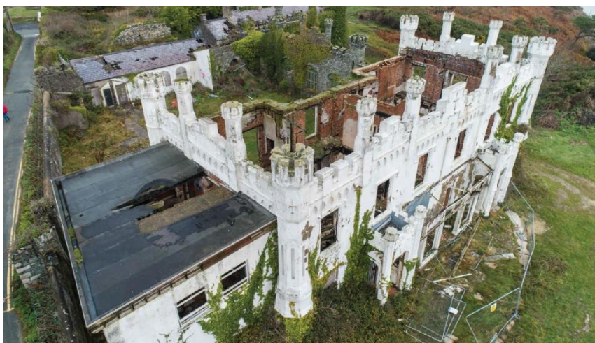
Aerial view of Soldier's Point House, demonstrating its current state of disrepair
