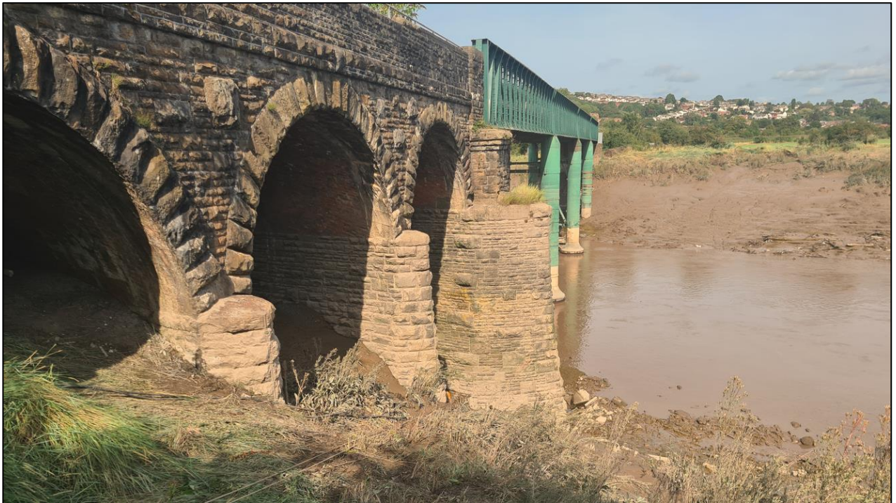
Figure 1: St Julian's Viaduct (Southern Shore – receding tide).
