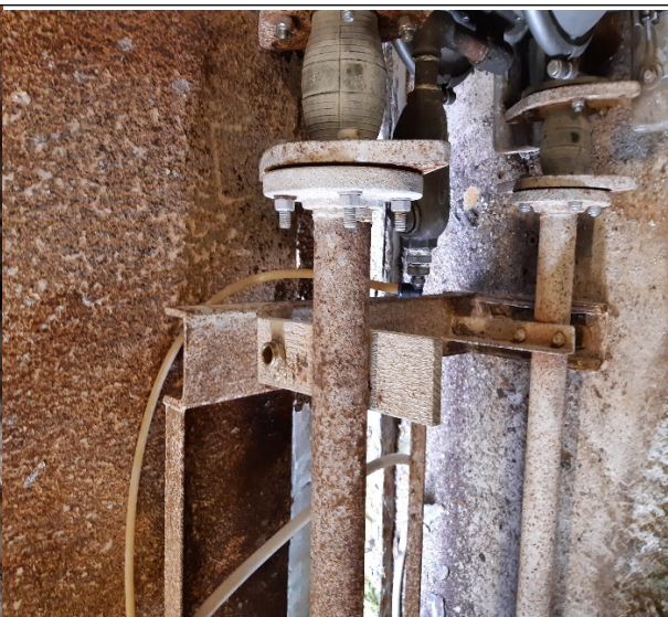
Image 5 - Corroded pipework
