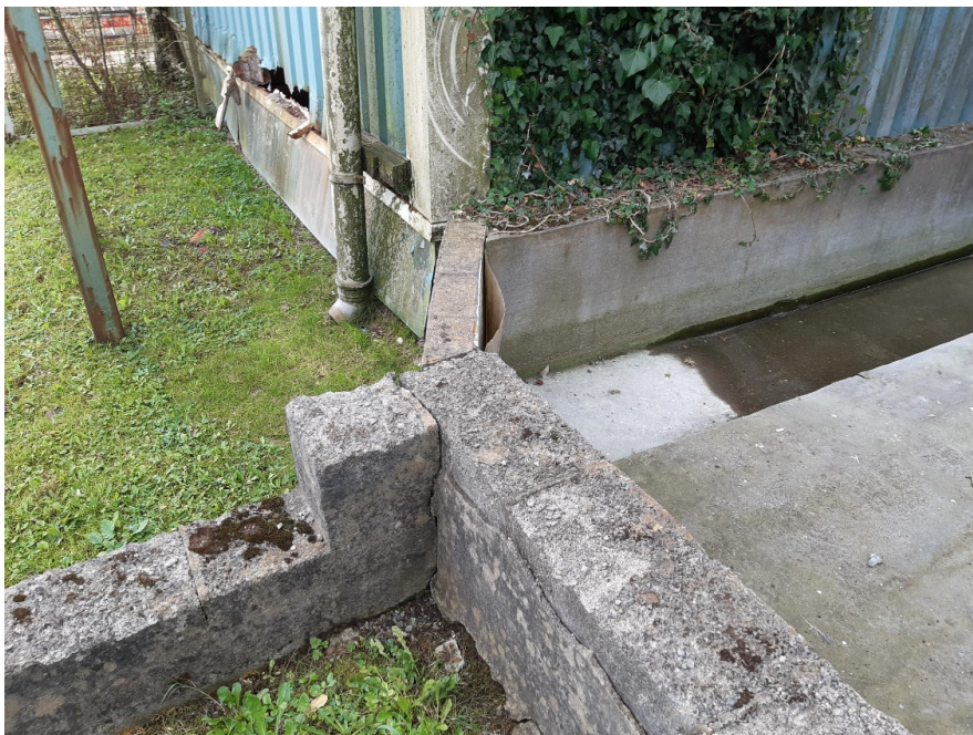
Image 8 – Bund walls not cast in situ and joint separation, block wall and render damage
