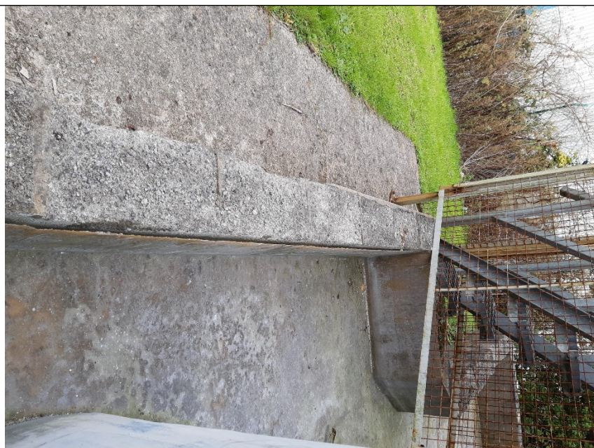
Image 9 – Fibreglass lining separation from bund wall.
