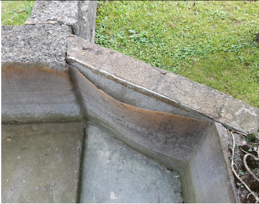
Image 7 – Wall joint and fibreglass lining separation
