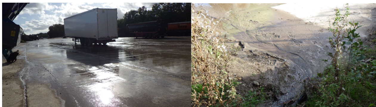
Photo left; looking towards the permitted area where dampening down had been taken place. Right; location where water was seen to be running off impermeable area.
