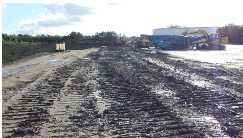
Photo taken of plant machinery moving the waste soil towards the quarry void, fresh soil can be seen within the quarry void.
