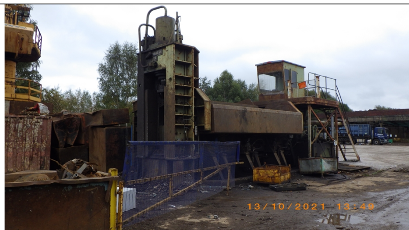
Photo to show crusher/shearer and newly gravelled surface adjacent
