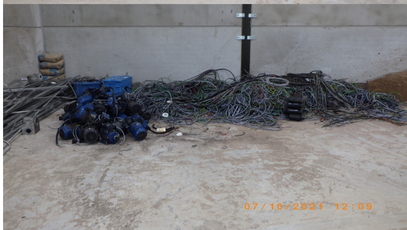
Photos showing waste storage inside the new transfer building
