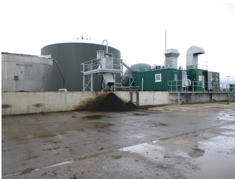
Image 2: Digestate removed from the digester
