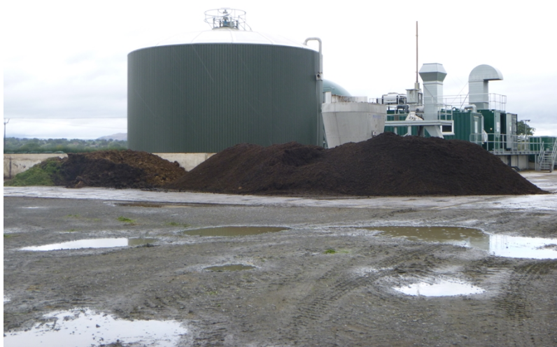
Image 1: Feedstock (left) and digestate (right) stored outside the AD Plant bund
