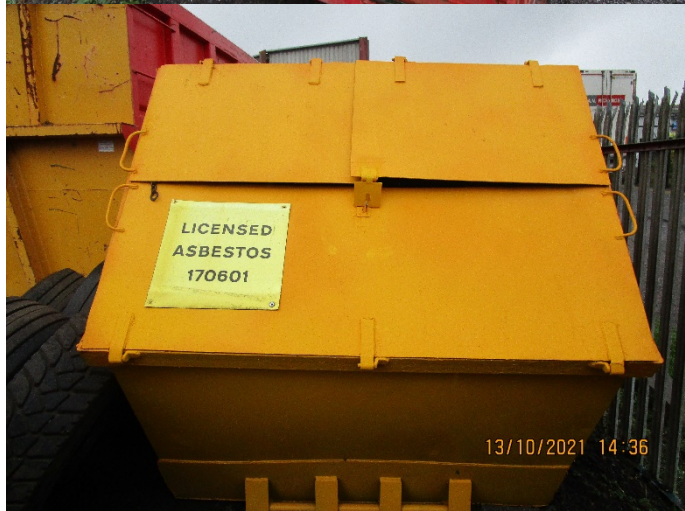
Figure 1. Labelled and separate lockable skips to store asbestos.
