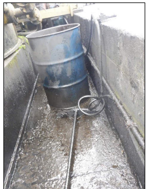
Photograph 6 & 7. Waste storage/treatment area. Secondary containment area floor in fair condition with some evidence of cracking.
