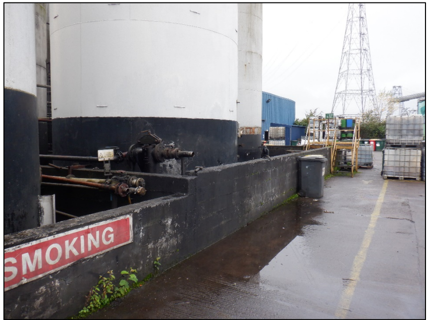
Photograph 4 & 5. Waste storage/treatment area. Breeze-block constructed secondary containment bund in poor condition.
