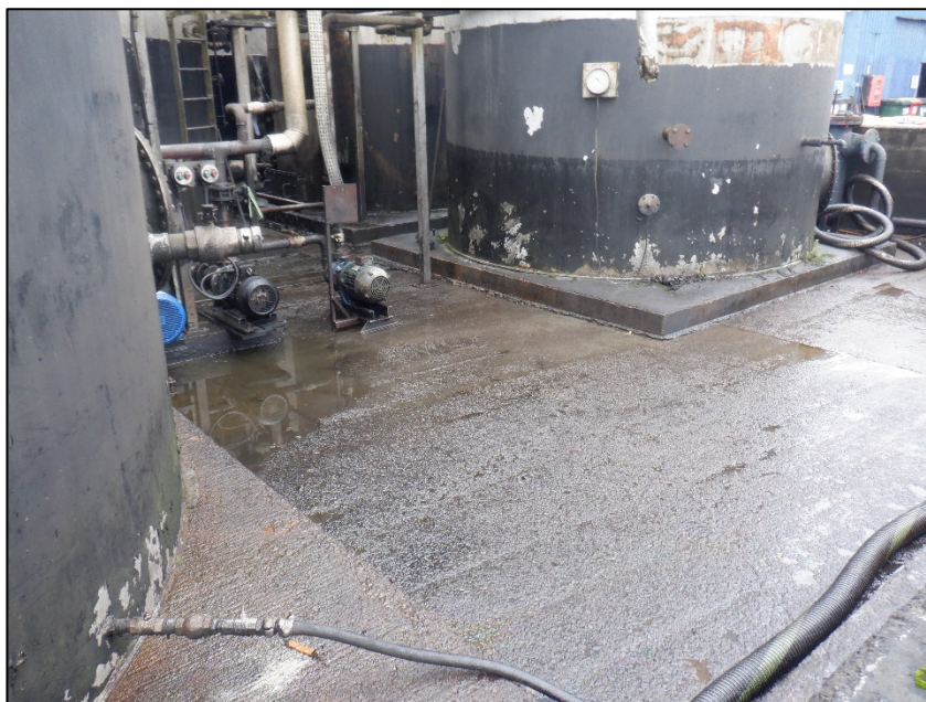
Photograph 6 & 7. Waste storage/treatment area. Secondary containment area floor in fair condition with some evidence of cracking.
