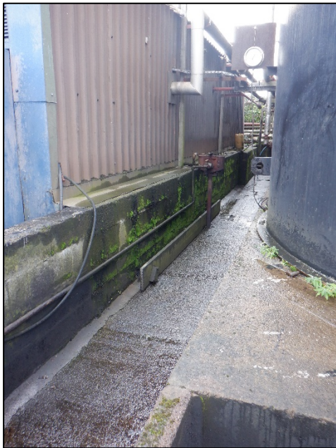
Photograph 4 & 5. Waste storage/treatment area. Breeze-block constructed secondary containment bund in poor condition.
