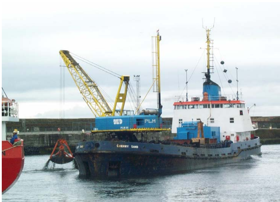
Plate 5. Grab hopper dredger “Cherry Sand” working inside a dock
