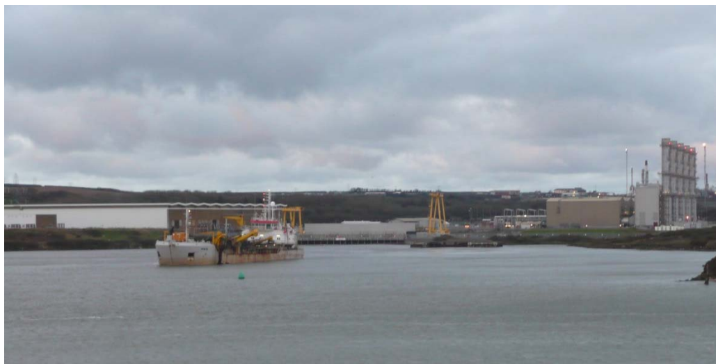
Plate 3. TSHD 'Pinta' dredging in Powerstation intake channel in January 2016.
