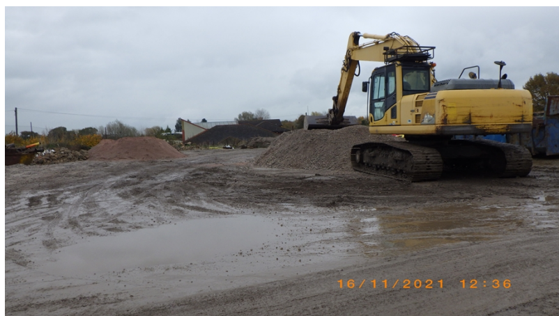
Photo showing area used to store incoming product such as sand and stone
