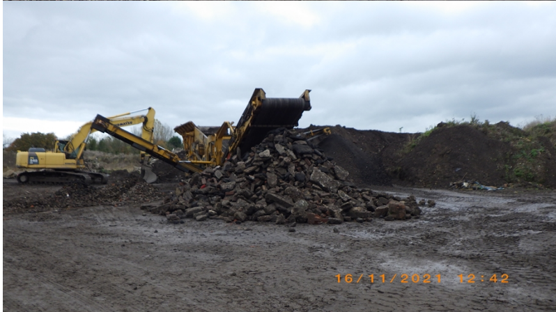
Photos showing machinery on site (crusher and screener)
