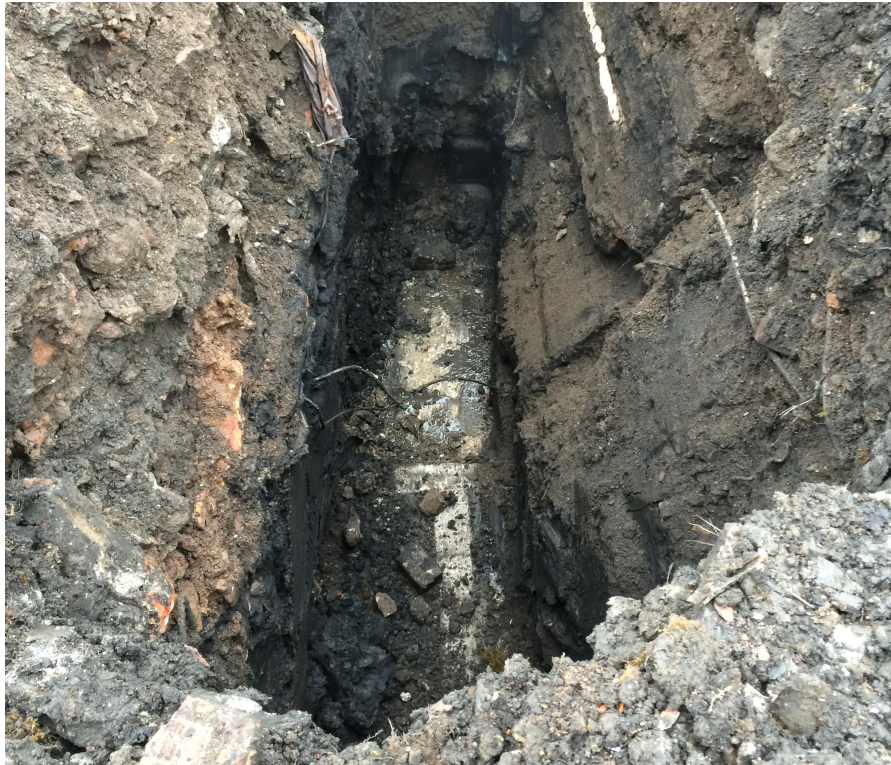
Insert 4: Subsurface concrete slab observed striking north south at 3m depth (Tp2d)
