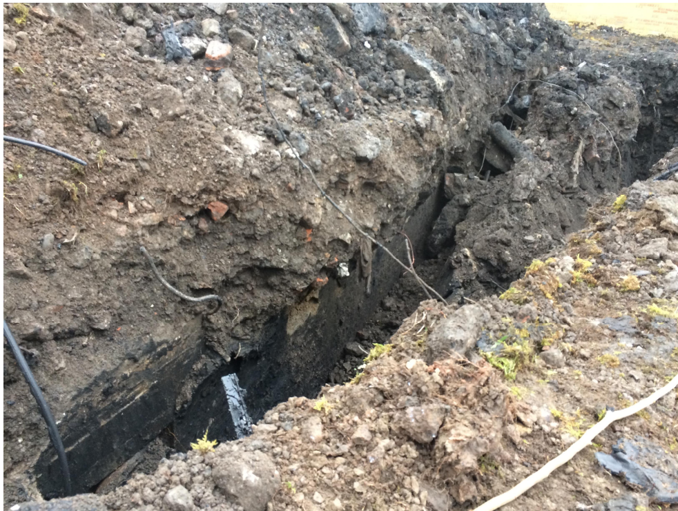
Insert 5: Subsurface concrete wall observed adjacent to 3m deep concrete slab striking roughly north south in the centre of the site. Note. The Made Ground has peeled from the wall.
