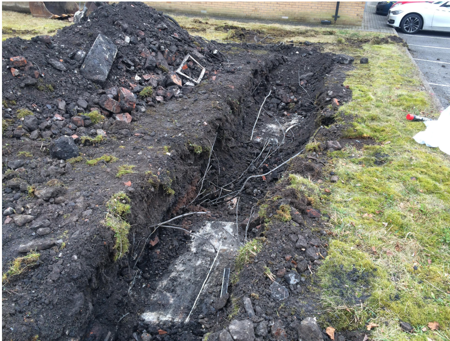
Insert 3: 2no. Subsurface Slabs with re-bar. Image taken looking South over TP1c
