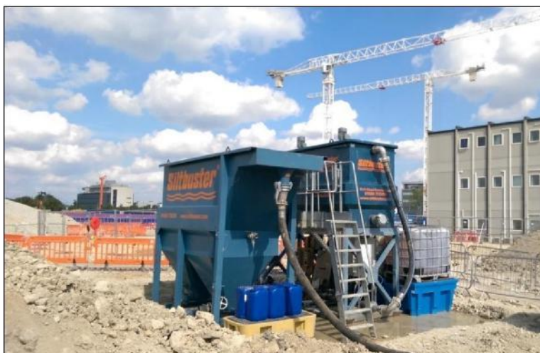
Figure 5 – Example of a 4 – 40m 3 /h, 2 Stage Chemical Treatment System (Mix Tank set up)
